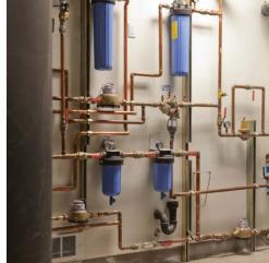
Photos Left to Right: Permitted potable rain water system – the first in King County, Installed photovoltaic system will produce much of the home's power, Solar pre-heating water system.
